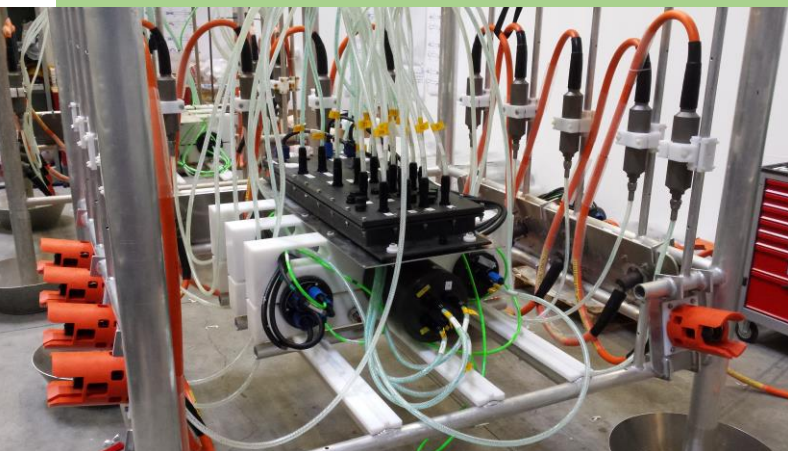
Phase-1 Junction box
