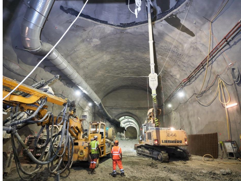
Civil engineering work underway for the HL-LHC
