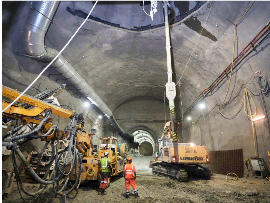
Civil engineering work underway for the HL-LHC
