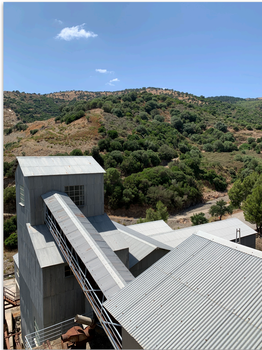
Former mineral processing unit
